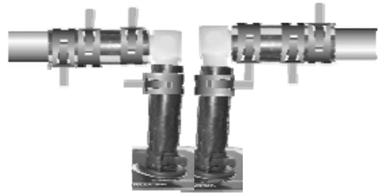
90° Connection Components Installed
