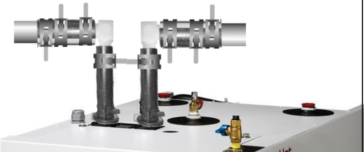
90° Connection Components Installed
