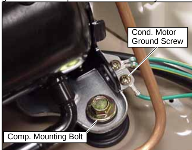
Figure 3-33 Condenser Motor Ground
