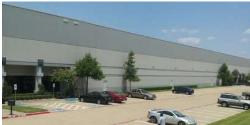
The Dallas distribution center
