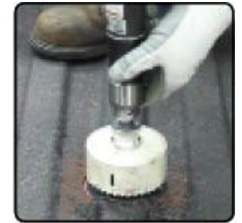
Use the pilot hole for error-free drilling
