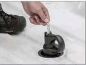
Step 4 - Secure with the provided linchpins
