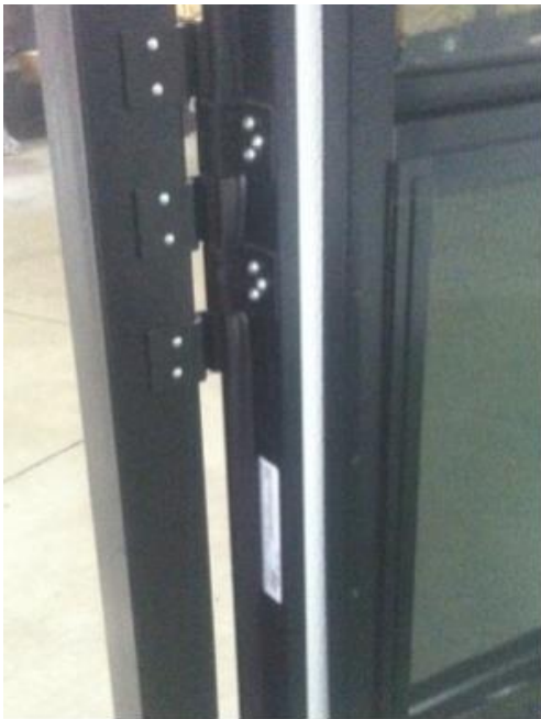
Entry Door Tag: Placed on the hinge side of the inner door frame and is only visible when the door is fully open. (Pictured Left)
