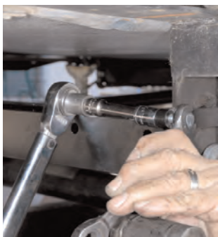
Install and torque the crossmember bolts.
